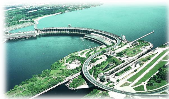
Fig.3 The Dnipro hydro development
