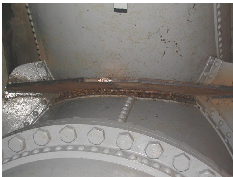
New reinforcement collar (rib).
