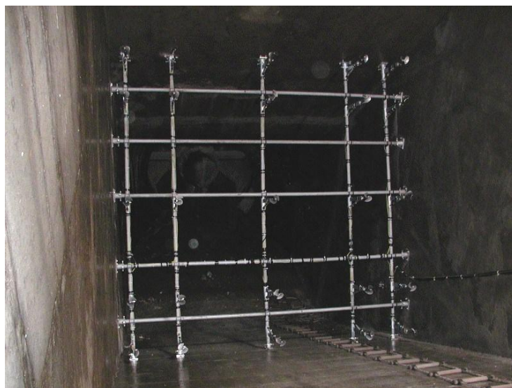
Fig. 9b Hydrometric section with the supporting frame and installed current-meters
