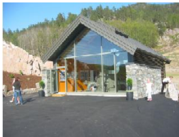
Figure 2 Oftedal Small Hydro Power Plant (Norway) 2006
