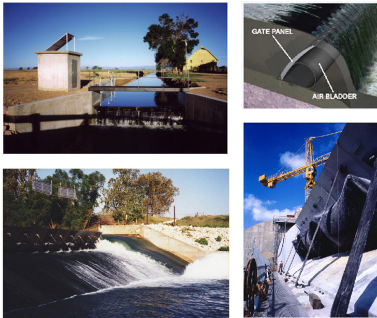
Figure 4 Pneumatic operated Spill Gates forming the dam
