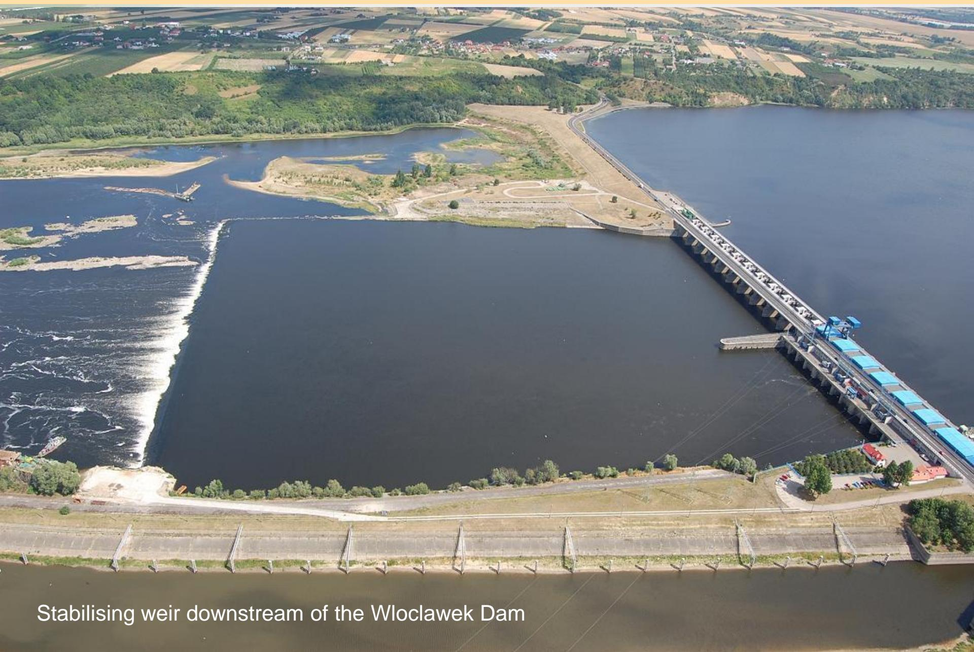
Stabilising weir downstream of the Włocławek Dam
